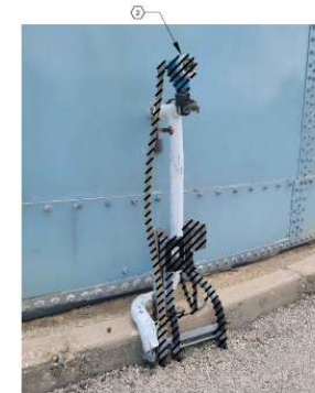
E EXISTING TANK LEVEL INSTRUMENT SCALE: NTS
